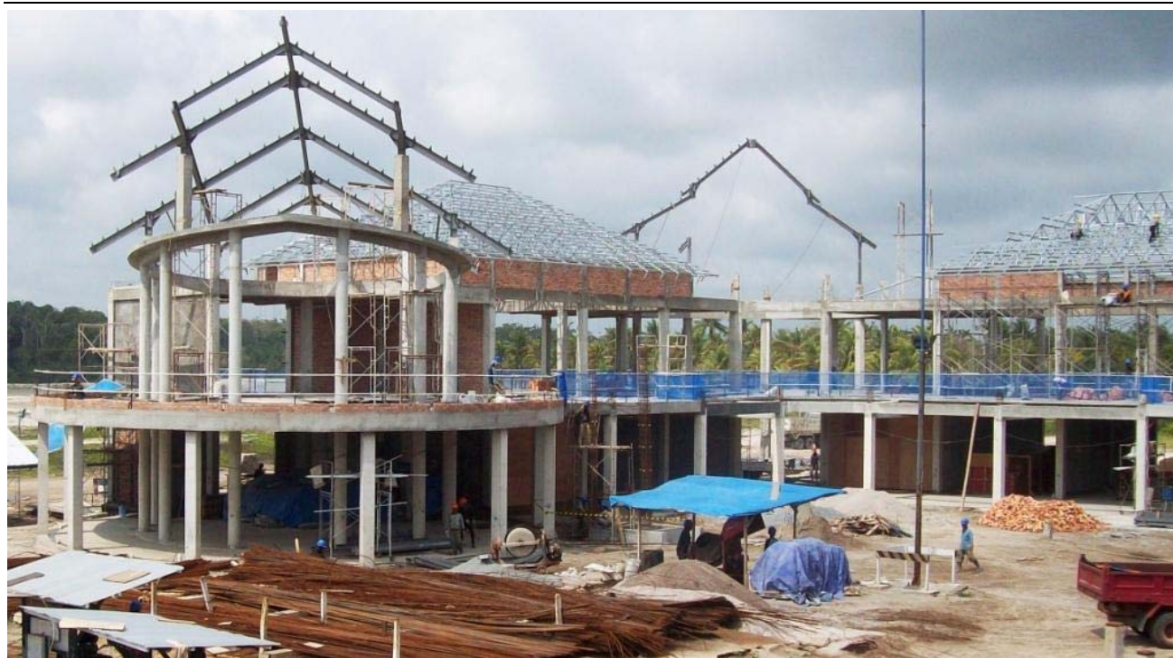
Figure 3: Lagoi Bay mall under construction
