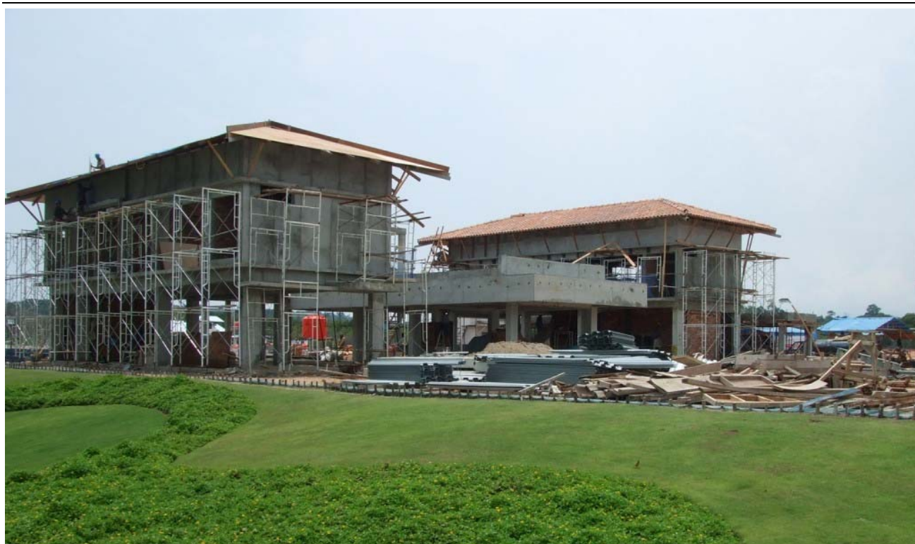
Figure 4: Ongoing work for Pantai Indah project
