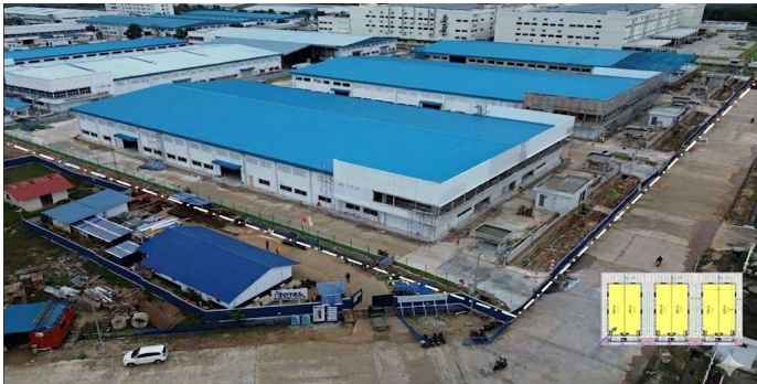
Ongoing new factory development in BIP to meet tenant demand
